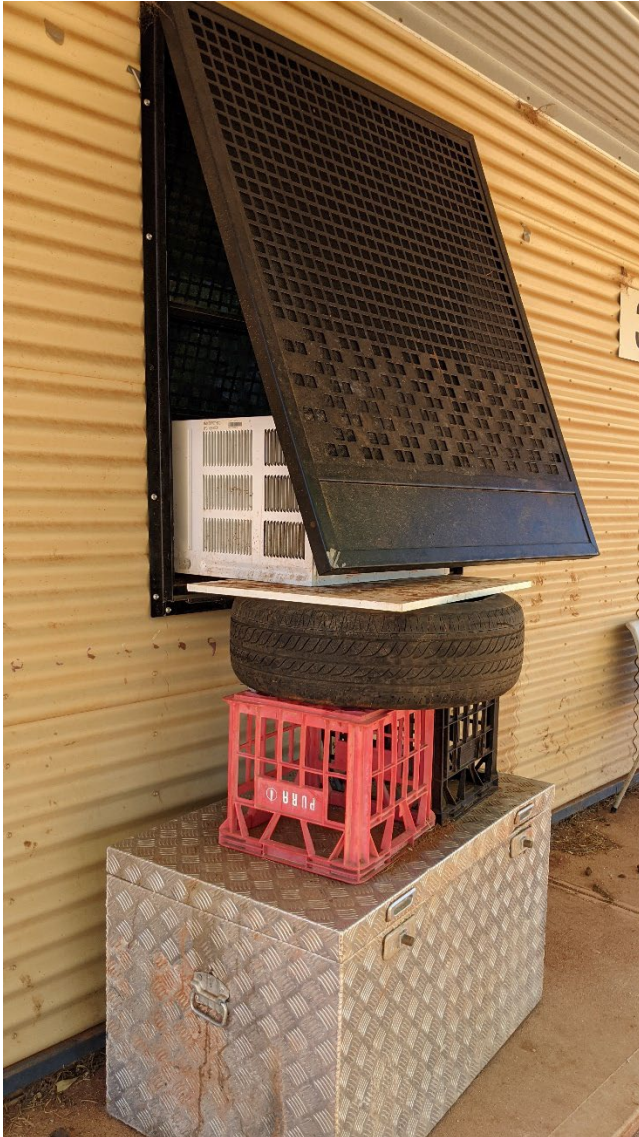
Figure 4. A precariously installed refrigerated air conditioner, below a security screen. Image: Liam Greal 2021.
