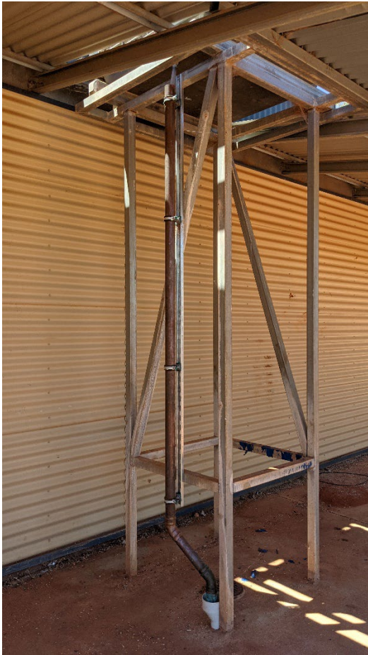
Figure 3. A water intensive evaporative cooler set adjacent to the house. This mode of cooling becomes relatively ineffective at high temperatures and high relative humidity. Image: Liam Grealay 2021.
