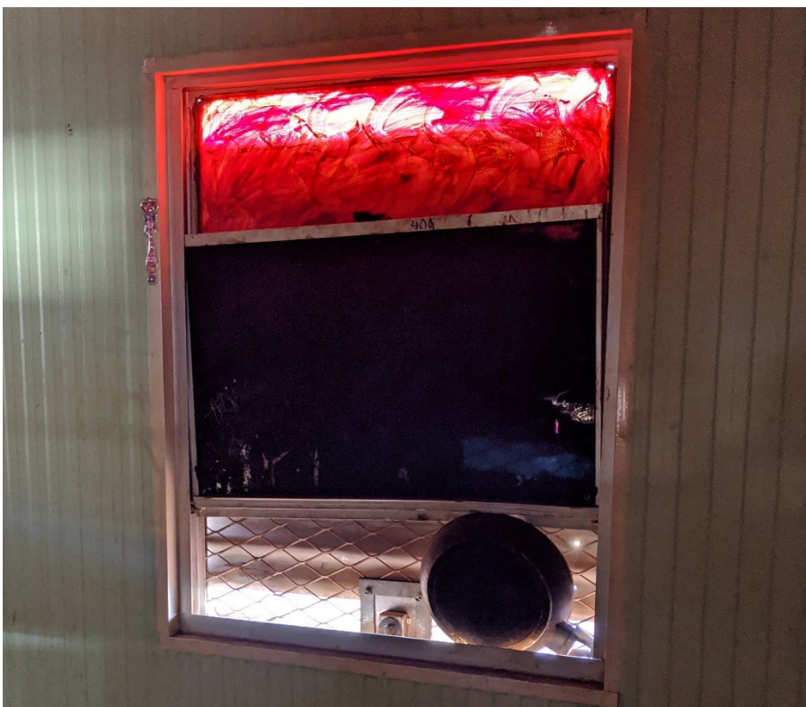
Figure 5. Window painted to reduce heat. Image: Liam Grealy 2021.
