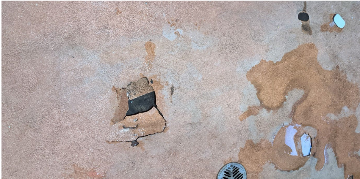
Figure 5: Bathroom floor at AACAP house in Pukatja. Image: Liam Grealty [Alt text: Deteriorated bathroom floor vinyl laminate and pooling water]
